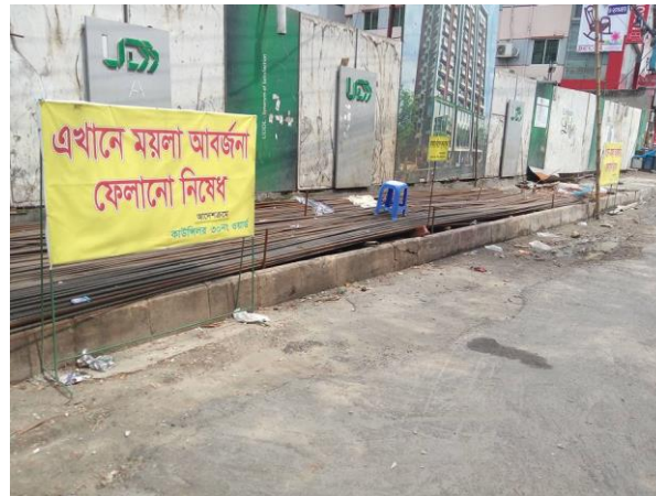
Photo 2 Construction Material and waste on footpath
