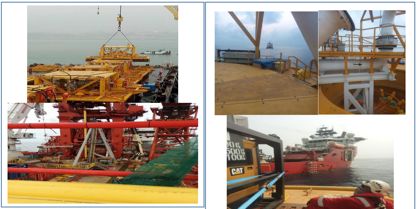
Figure SEQ Figure \* ARABIC 75: Images on the left depicting operations prior to subsea development offshore; thus image of FLETs onboard by Polar Onyx crane in Takoradi Port prior to departure for Sankofa field in 2017, and Lewek Constellation with flex pipelay unspooling from aft rail heading over TLS tower amidships and down the Moonpool to subsea on the Sankofa field ; and Images on the right shows the 2020 Jubilee turret buoy installation being anchored to the seabed with the aid of AHTS Skandi Skansen), tug, Seven Adaba and Bear
