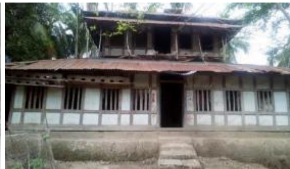
Figure 6.37: Two-story traditional houses as protection against the tidal surges.
