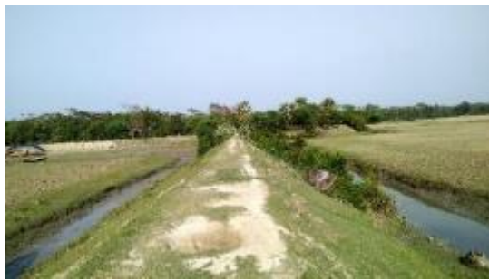
Flood protecting embankment at Patharghata (Zone-A)
