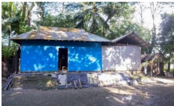
Figure 4.21: Migrant people built their houses on the extension of an existing homestead.
