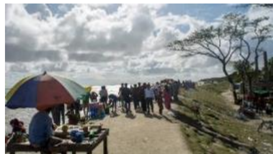
Erosion protecting embankment at Ramgati (Zone-B)
