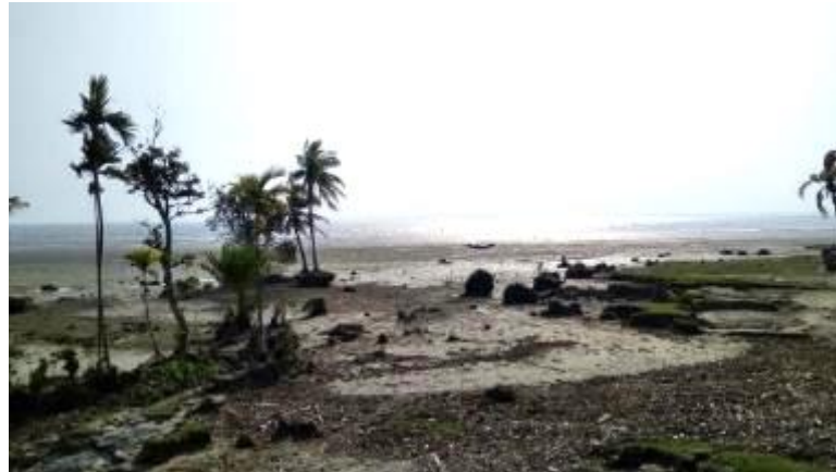
Figure 6.26: Settlements were washed away by Sidr in 2007 in many areas of Zone-A.
