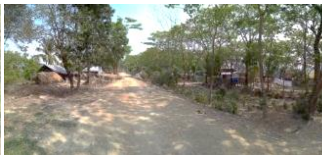
Figure 4.17: Settlement of Char Duani along with the embankment.
