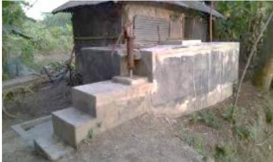
Figure 6.30: Filter to make the pond water drinkable
