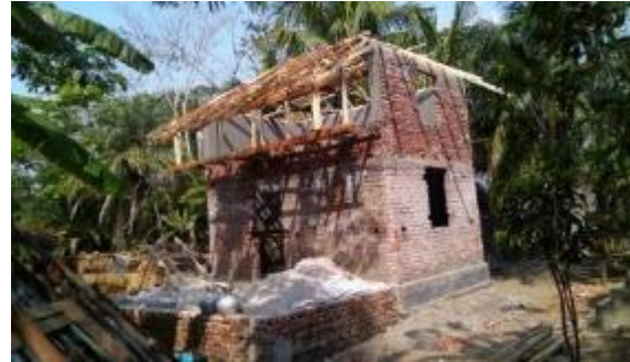
Figure 6.31: People are making small buildings with permanent building materials in Padma Char of Zone-A.
