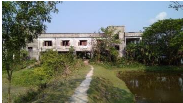
Figure 6.23: Cyclone Shelter Centre at Patharghata (Zone-A)
