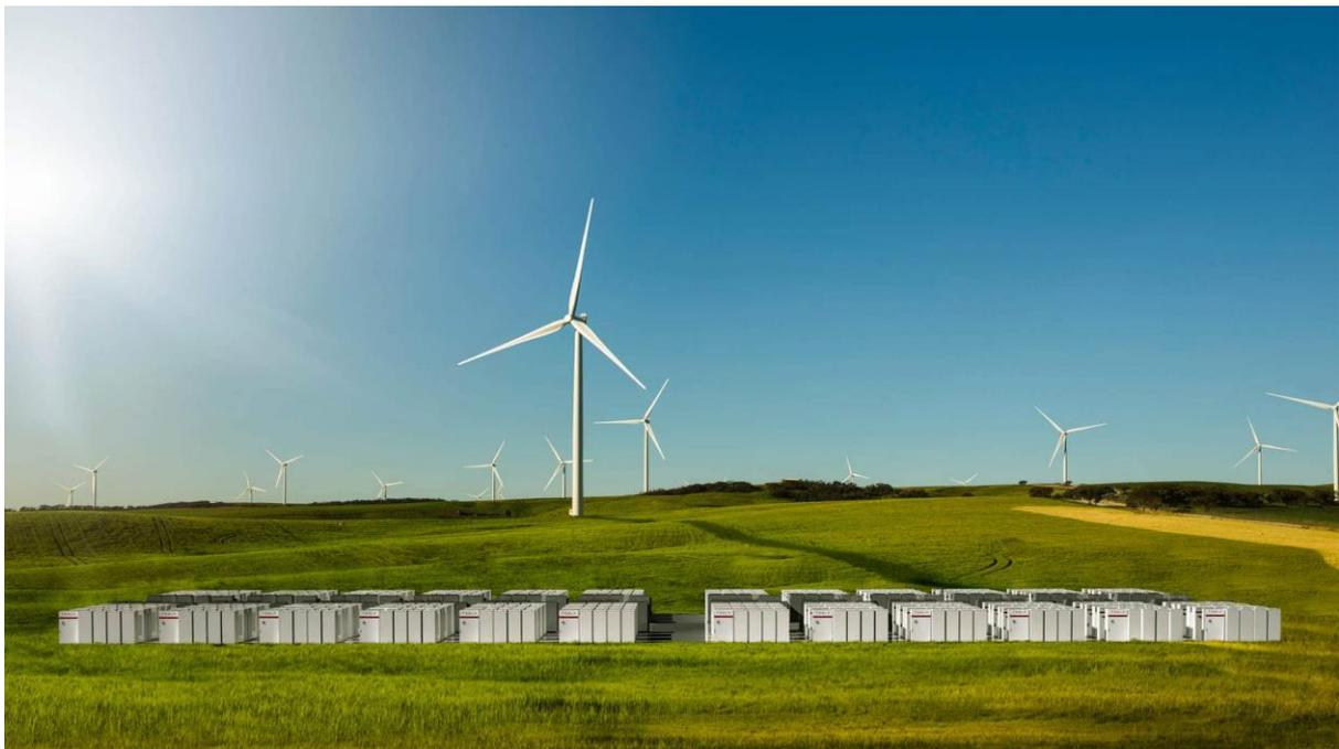
*Figure 13. Tesla 100 MW/ 129 MWh Li-ion battery storage installation at the Hornsdale wind farm, Australia.*
