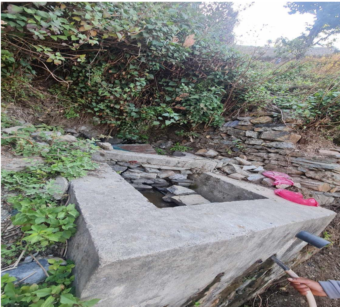
Figure 9 Dam/ Intake ready for improvement
